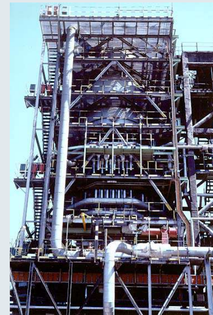
SASOL - Slurry phase distillate reactor 1)
